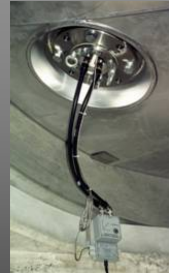
Insertion Sensors Installation below a pan
