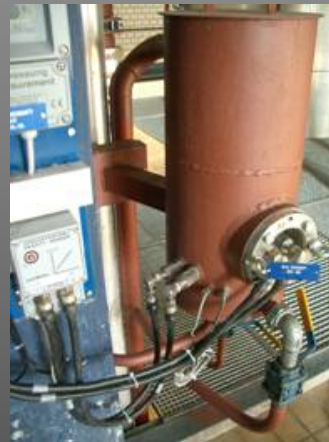
Rod Sensors Direct mounting in a boiler
